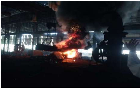
Work zone with Canopy Hood
