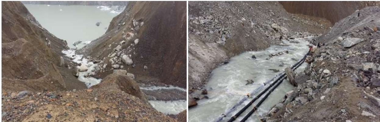
I. Photograph showing the stream draining to the South Lhonak lake & II. The photograph showing laying of pipelines with the help of rope in September 2016
