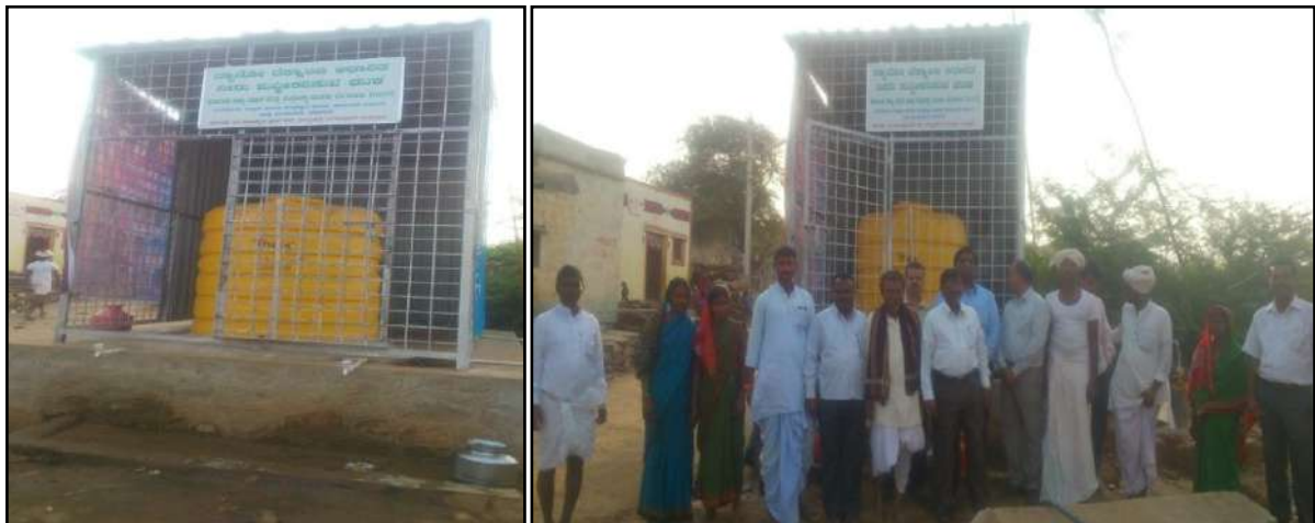
Nano Tehnology based water purifying unit at Hal Ammapur village,Shorapur taluk, Yadgir district
