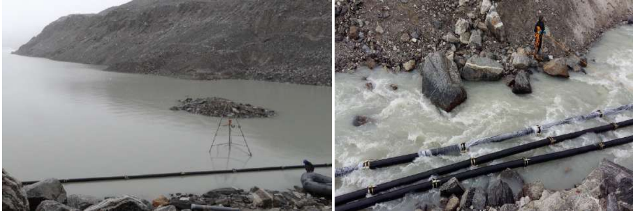
I. GLOF sensor installed in South Lhonak Lake & II. Pipelines laid down for the siphoning of water from South Lhonak Lake
