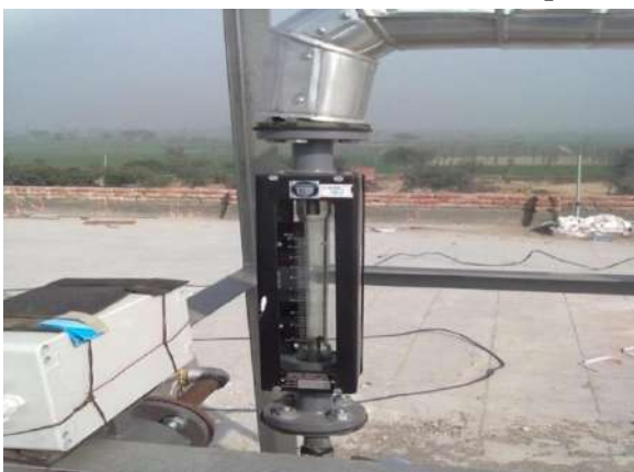
Rotameter for Thermal performance Test set-up
