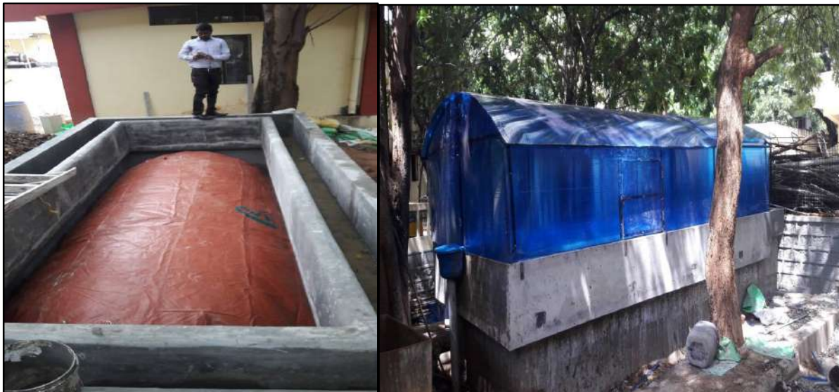
Bio-digester plant installed at CCMB
