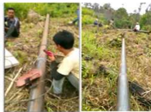
Work under Progress
