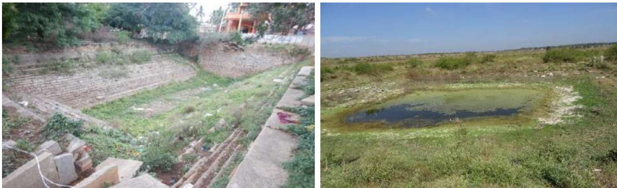
Kalyani in Doddaballapur, Doddaballapur Tq, Bengaluru Rural District
