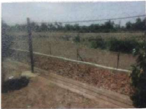
Chain Link Fencing
