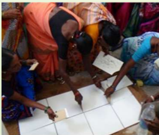
Training on Tiles Grouting
